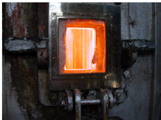
A window of heating furnace
